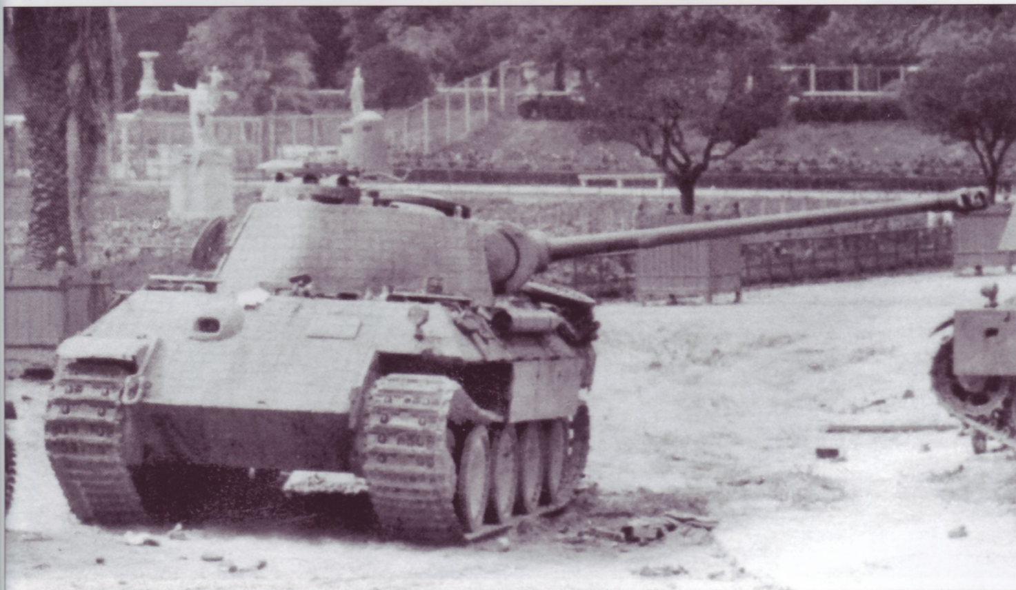
A pair of abandoned Panthers as well as another tracked vehicle litter a road, which, by the looks of the statues, fountains and trees, could be somewhere in Italy. The Panther in the center of the photograph is an Ausf.A, readily identified by the MG ball mount and the open driver's visor on the upper glacis plate. It is covered in Zimmerit and still wears most of its Schürzen. It is finished in a monochrome coat of dunkelgelb and carries no visible markings. Note the spare road wheels on the turret roof and engine deck.
