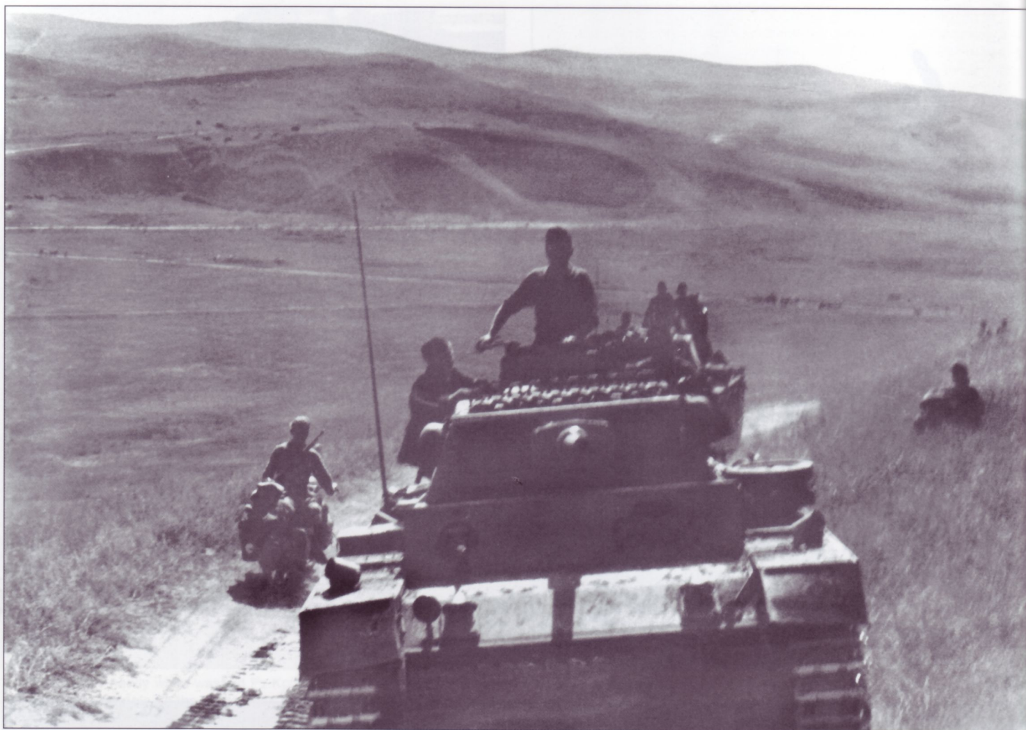
This Pz.Kpfw.III Ausf.J or L has the frame for additional spaced armor on the mantle, but the armor itself has not been fitted, due to production shortfalls. That on the superstructure front has been fitted. This particular panzer is unique in that it has what appear to be either S-mine or smoke dischargers mounted on each fender, just behind the mud flaps. There also seems to be a third discharger mounted just forward of the rod antenna.
