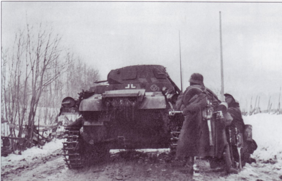
A column of Pz.Kpfw.III (Ausf.D, E or F) leads a Pz.Kpfw.I Ausf. B ohne Aufbau, which has been converted into a vehicle to carry maintenance equipment for the panzer company's repair and recovery sections, by the removal of its superstructure and turret. It was also known as "Instandsetzungskraftwagen I". Note the yellow gothic "I" (which appears to be a "J") that identifies the vehicle's function, on the rear corner of the engine deck, as well as the white "K" of Panzergruppe von Kleist. Note also the small square tactical markings on the rear turret face of the Pz.Kpfw.IIIs and the racks for jerry cans on their rear decks.
