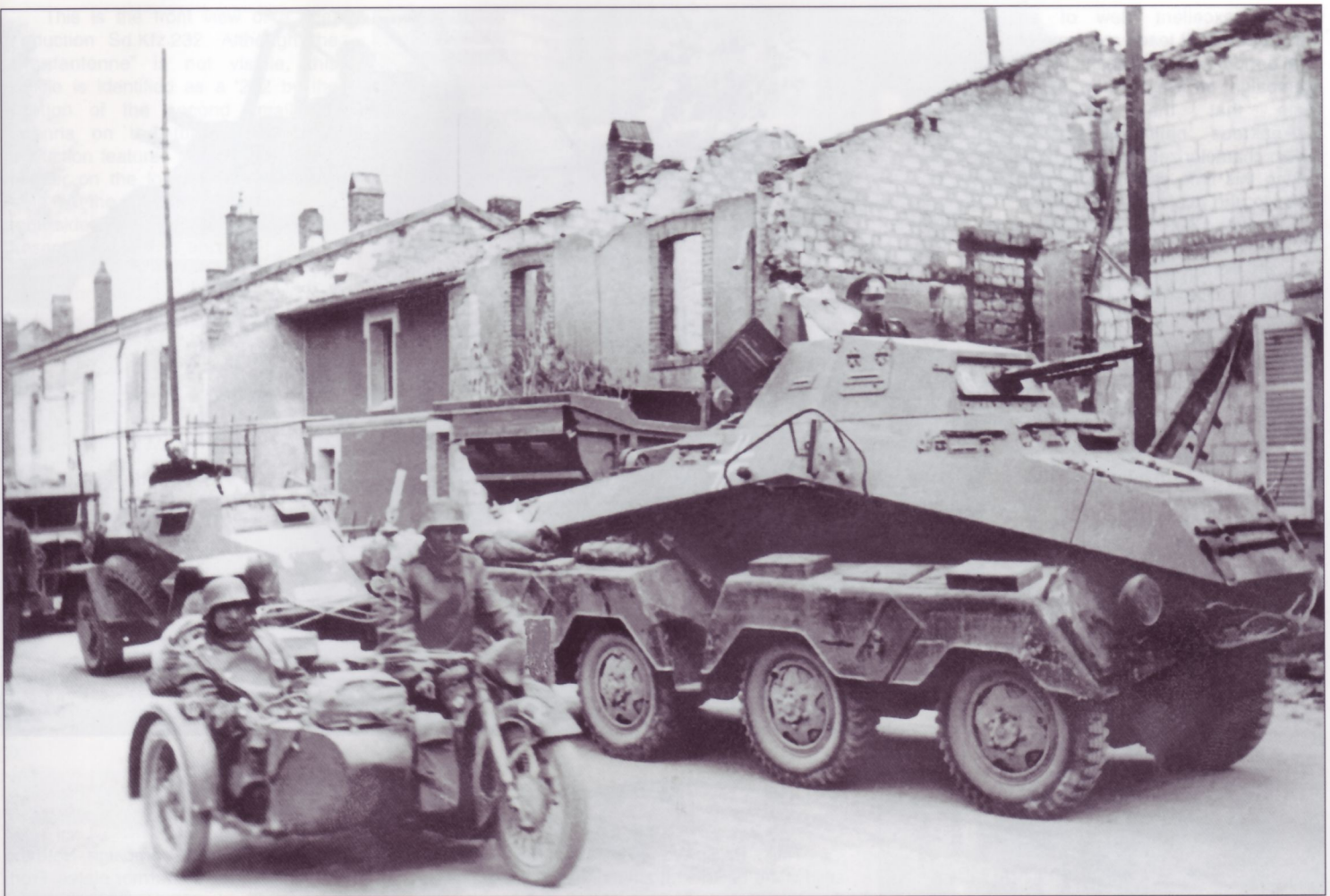
An Sd.Kfz.231 (8-rad) leads an Sd.Kfz.223 through a shattered town, probably during the French Campaign in 1940. They are accompanied by a heavy motorcycle combination based on the BMW R75. All the vehicles are heavily covered in dust, which makes the base colors appear much lighter than they actually were, due to the way light is reflected. The sole markings visible are a white-outline balkenkreuz on the '231 and a Tac sign on the R75.
